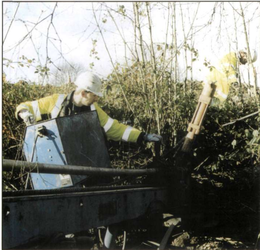
Figure 6 Horizontal drilling being used for laying a cable under a road
