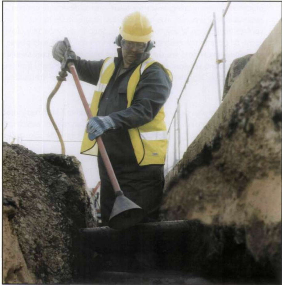
Figure 5 Using an air digging tool
