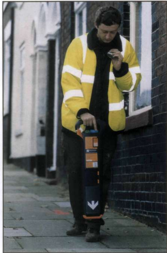
Figure 4 Using a cable locator
