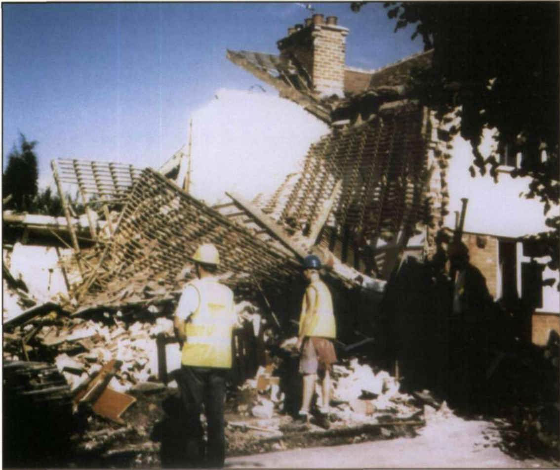
Figure 1 Aftermath of a gas explosion, following damage to an underground gas service pipe
